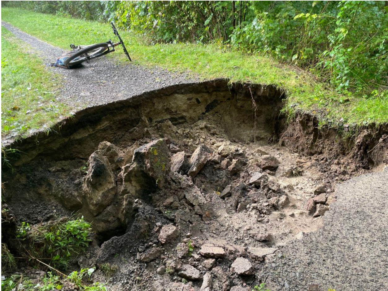
Sinkhole on Hojack Trail near Drumm after Rain Event MO 9/9 (Ben W. photo)
